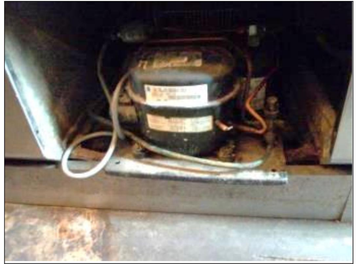
50. Interior bar area; Stainless steel ice cream cooler refrigeration unit to remain
