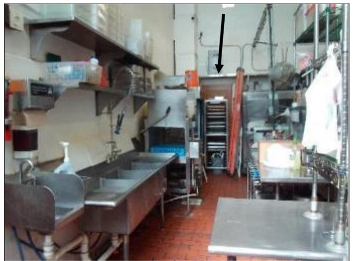
72. Overview of the kitchen area; Note the locked access door leading to the west adjoining TRE meeting room
