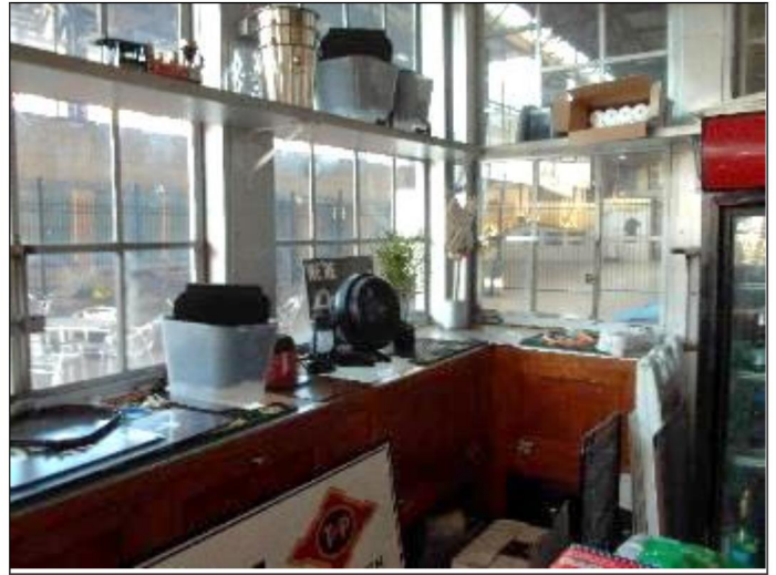
44. Service/bar kiosk shelving and cabinetry to remain
