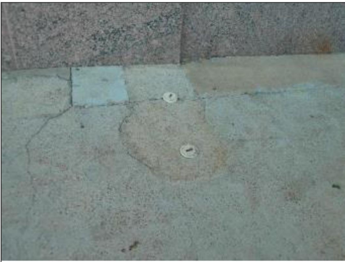
9. PVC sanitary cleanouts for the building sewer system
