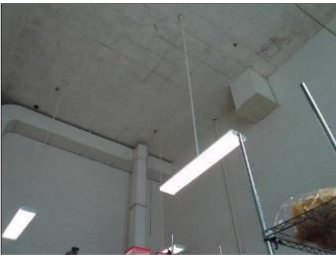
71. Kitchen ceiling finishes and suspended LED lighting fixtures
