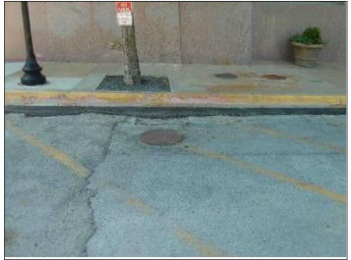
8. Location of the sub-grade sanitary sewer connection to the Municipal sewer system
