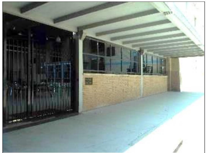
4. East façade and canopy at the south exterior patio area
