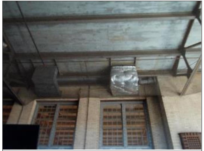
64. RTU ducting conditions
