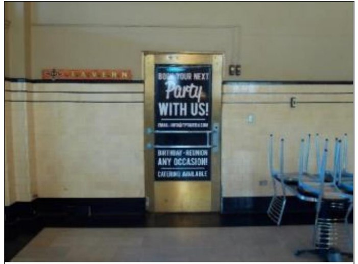
68. Dining/bar area locked access door leading to the west adjoining TRE Function Hall
