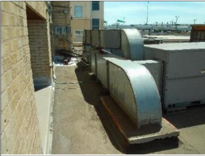
63. RTU ducting conditions
