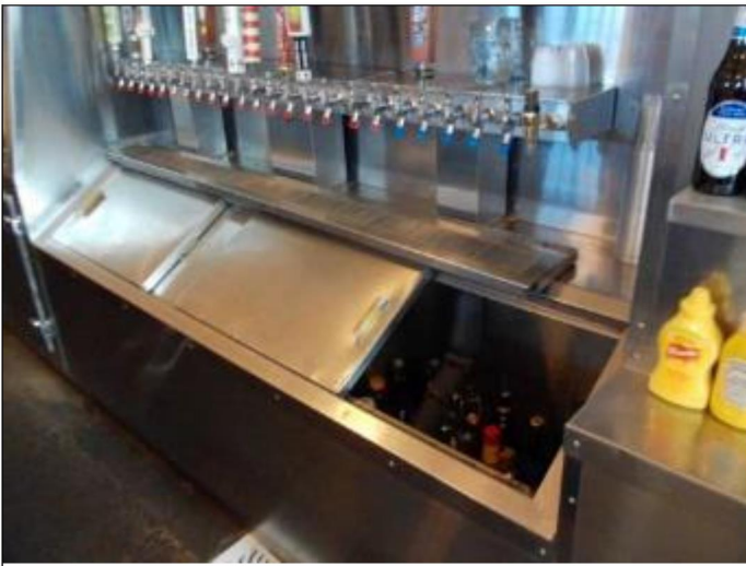
51. Interior bar area; Stainless steel beer cooler to remain
