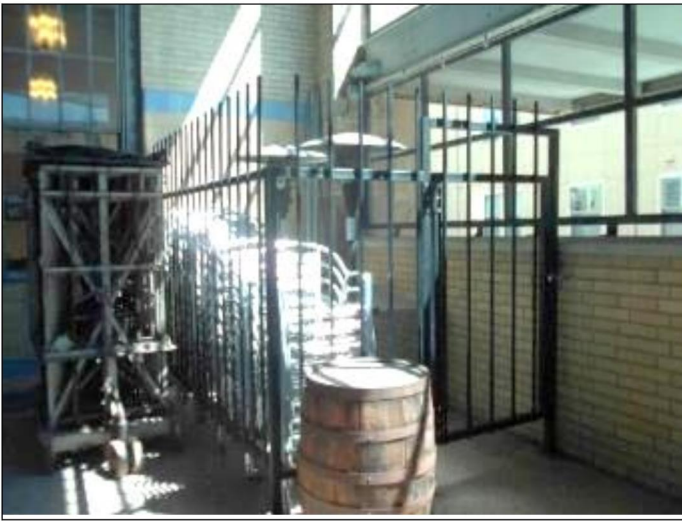
39. South exterior patio area storage cage structure to remain
