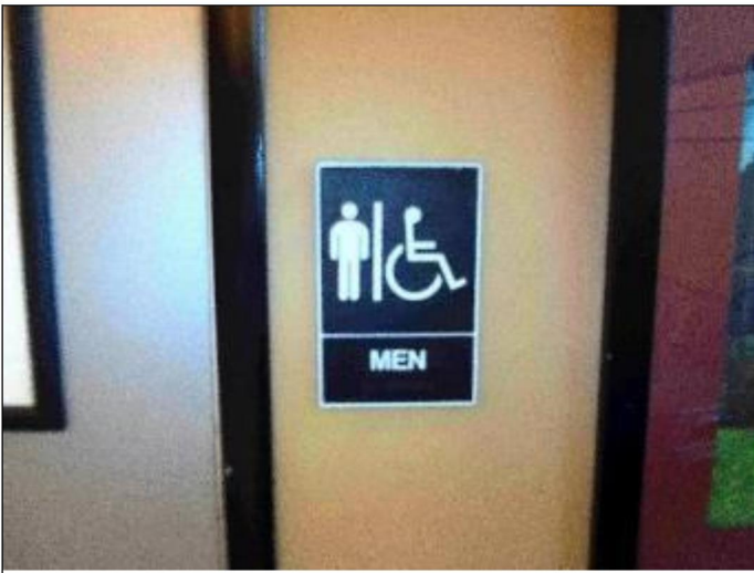
57. The restroom signage is missing compliant signage (Braille lettering is missing)
