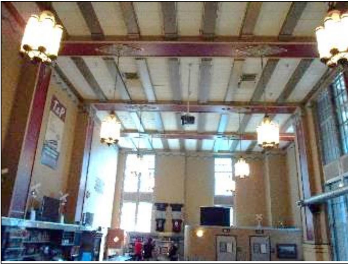
55. Dining/bar area chandeliers (8) to remain; Note chandeliers have LED bulbs
