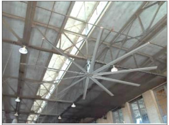
40. South exterior patio area 'Big Ass Fan' unit to remain; Note all patio area lighting is LED
