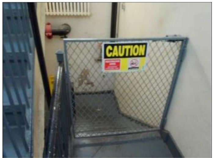
12. Basement access stairs and gate
