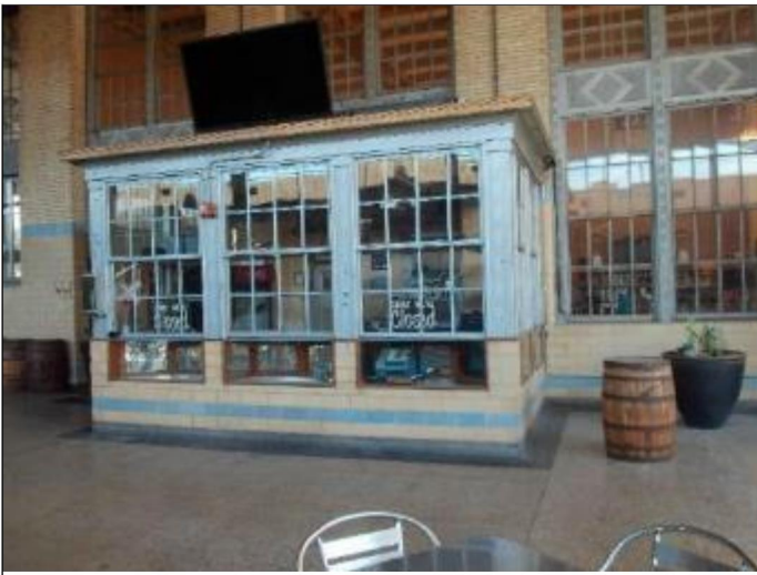
41. South exterior patio area service/bar kiosk to remain
